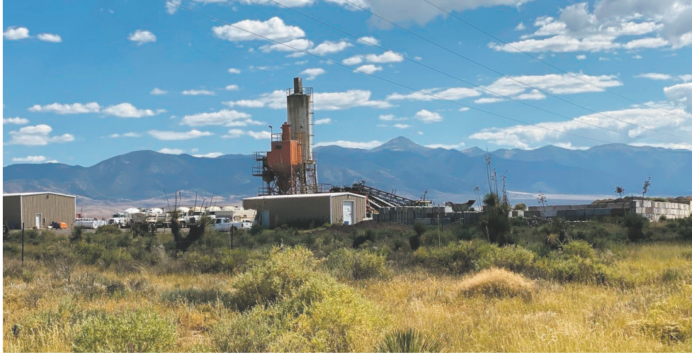
Above: The site of the proposed Roper concrete batch plant, with a nursery visible in the distance. Inset: The Roper plant in Carrizozo, N.M.
